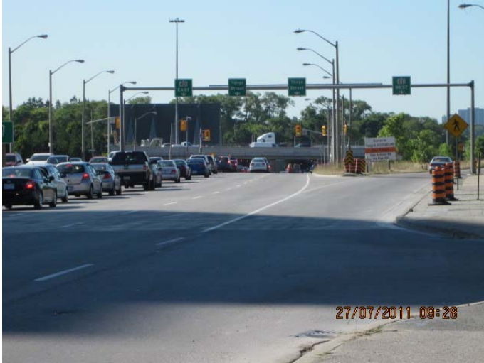
Photo 1: N-E 401 Left Turn “Waiting” Lane - Southbound Yonge Street to Eastbound Highway 401 on-ramp (N-E 401 on-ramp) left turn “waiting” queue in mid-morning. Notice, higher service volume right turn is clear without any queue.
